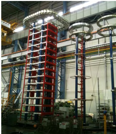
Modern Impulse test equipment
